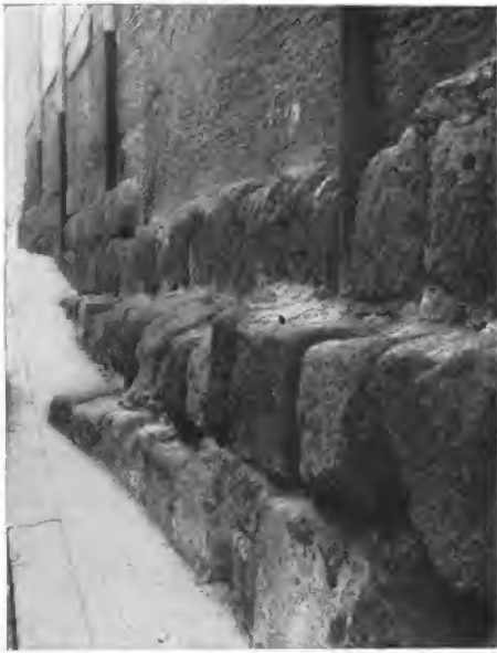
Fig. 96a. S. Martino ai Monti, Ninth century basilica, foundation and rising wall of east aisle
